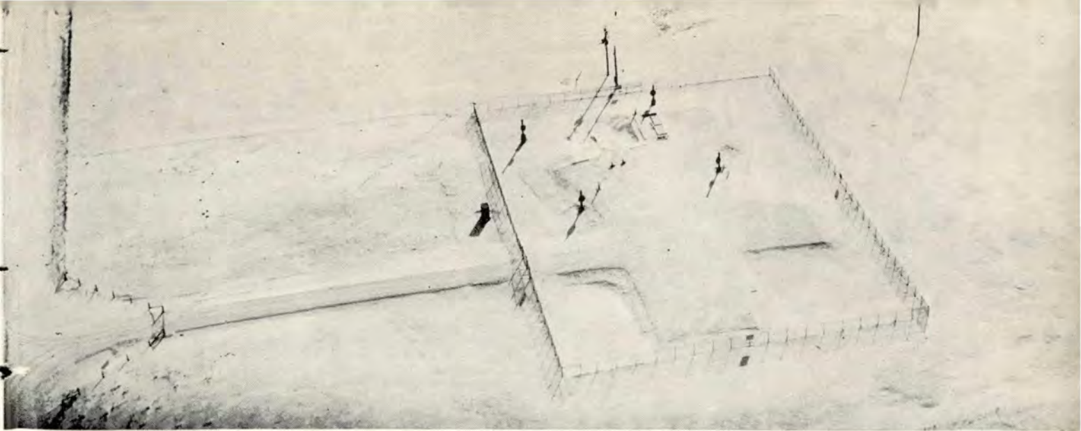
Like this Minuteman site, most missile launch facilities are located in a cold climate which presents a variety of safety problems for missilemen.
